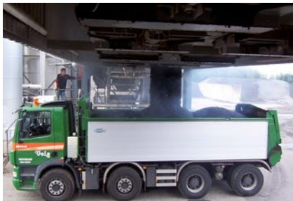
Asphalt and concrete mixing
